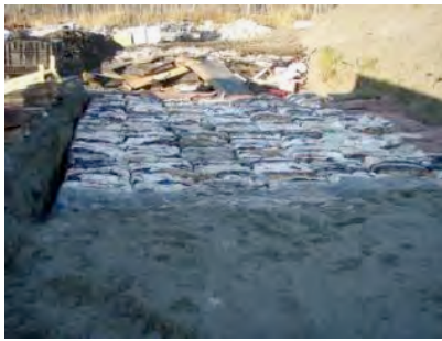
The trash bales in place.
