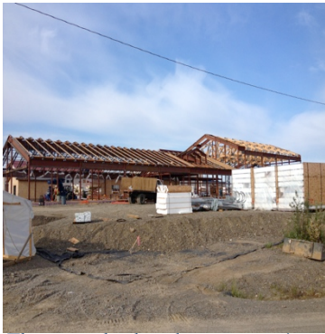
The new school under construction
