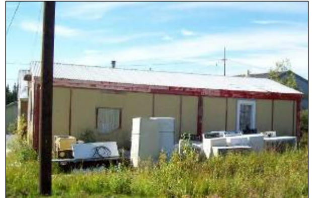
Kiana's temporary recycling center and appliance staging area.
