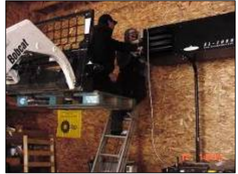
Selawik installs their used oil burner in their workshop.
