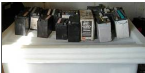
Collected lead acid batteries to be backhauled.
