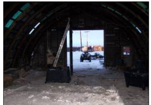
Akiachak is converting an old Quonset Hut into a hazardous waste staging and solid waste Reuse Center. They plan build up their Center to use for future regional staging and backhaul along the Kuskokwim with other villages.
