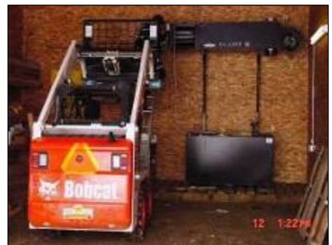
Selawik installs their used oil burner in their workshop.
