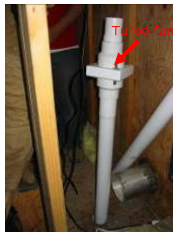
Fig 57: Vent pipe coming up from the bathroom in the attic space with the turbo fan attached with a 3" coupling
