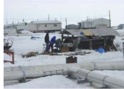
Figure 3: Above ground piping structure passing through the center of a community
