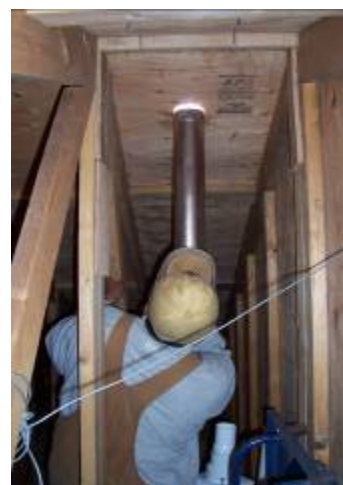
Fig 57: Vent pipe coming up from the bathroom in the attic space with the turbo fan attached with a 3" coupling
