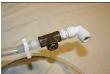
Figure 45: Close-up of pipe fitting which attaches to the drain outlet on the toilet
