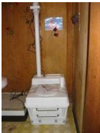
Fig 75: Installation of the Snow's toilet.
