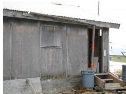
Figure 11: Household rain catchment system
