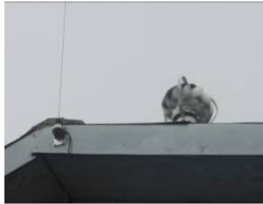
Fig 63: Mounting the satellite antenna to the roof
