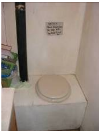
Fig 52: Honeybucket under a wooden bench and toilet seat in the store bathroom prior to compost toilet installation
