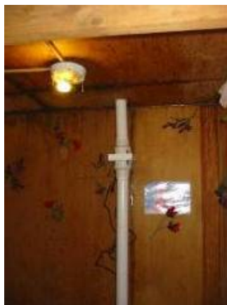
Fig 76: Lining up the vent pipe for the Snow's toilet.
