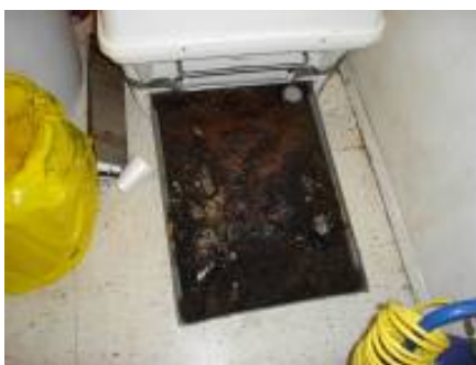
Figure 99: Full tray removed from the store toilet during emptying.
