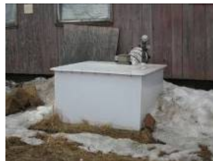
Figure 13: Flush-haul wastewater tank outside a home
