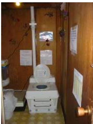
Fig 77: Snow's toilet installed with signs put up on the bathroom wall, door and toilet.
