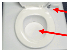
Figure 27: Handle and disk in closed position
