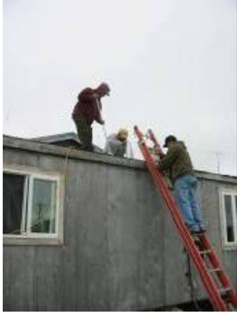
Fig 81: Working on the roof above the Snow's bathroom.
