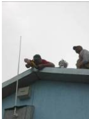
Figure 38: Installing the antenna to the roof of the store
