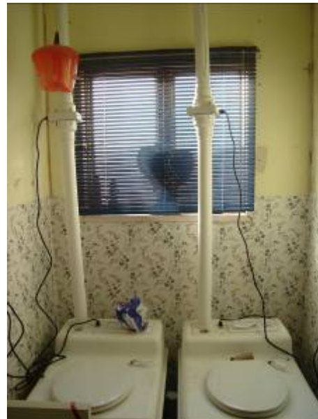
Fig 95: Toilets A and B installed and plugged in the Moss's bathroom.
