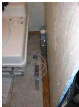
Fig 90: Modified drain pipe with container placed to the right of the Tundra's toilet.
