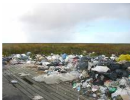
Figure 18: Another angle of the overflowing honeybucket lagoon and dilapidated boardwalk
