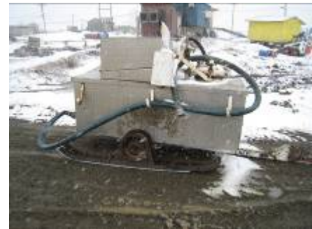
Figure 4: Above: Flush-haul wastewater tank outside a home. Figure 5: Below: Vacuum tanker used for removing wastewater from flush-haul systems
