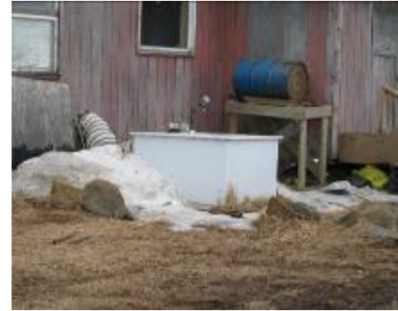
Figure 4: Above: Flush-haul wastewater tank outside a home. Figure 5: Below: Vacuum tanker used for removing wastewater from flush-haul systems
