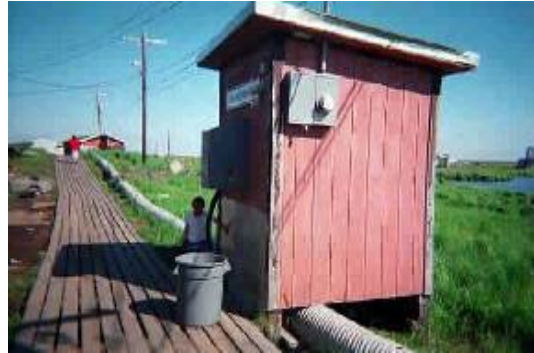
Figure 10: Public water dispensing location in Raven
